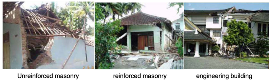
Fig. 4 Buildings damaged types (Daryono, 2011)
